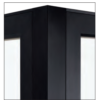
EXTERIOR CLOSE UP
